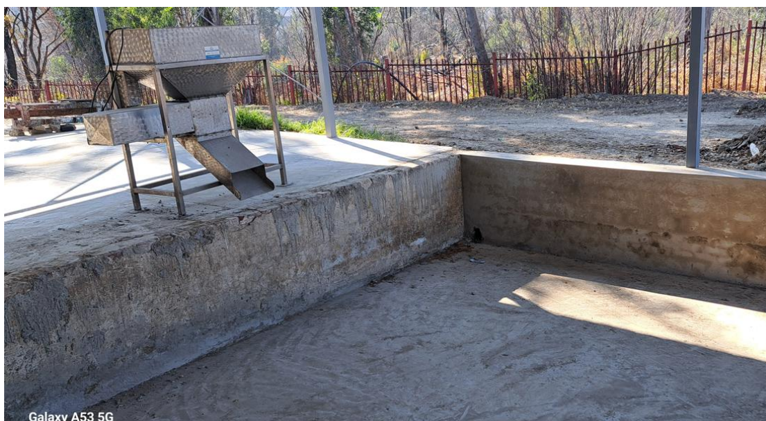
Photo 06: Hatchery wastewater screening unit and separation pit
