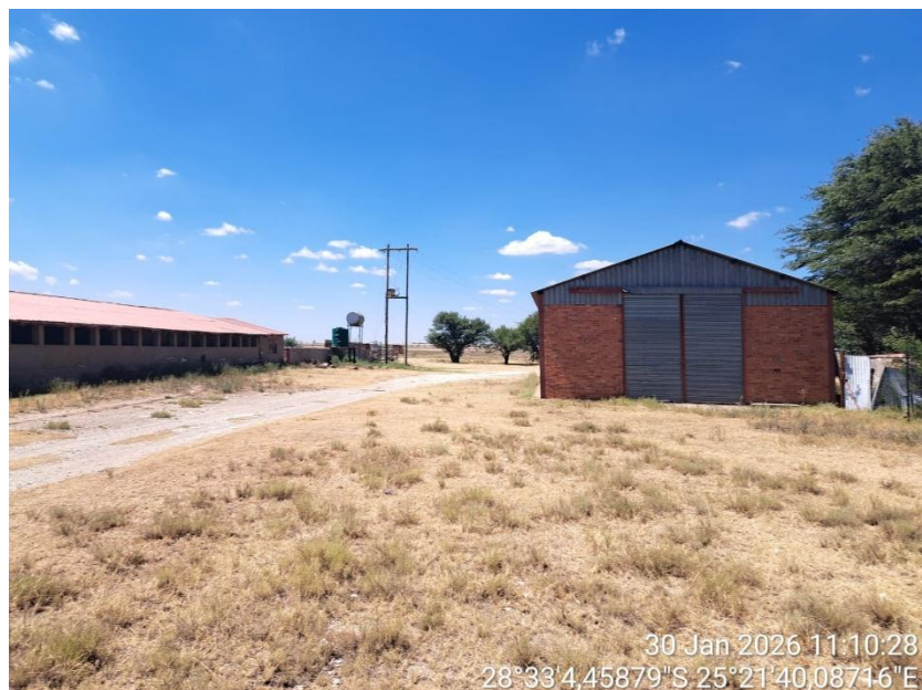
Existing farm infrastructure and electricity connection point
